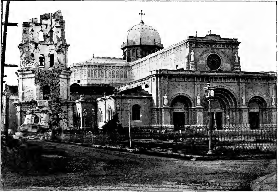
CATHEDRAL OF MANILA AFTER EARTHQUAKE.
